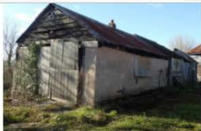
Figure 6. The southeast gable wall & northeast elevation of Barn 7
