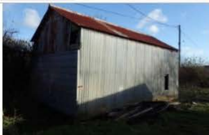
Figure 7. The northwest gable wall & southwest elevation of Barn 8
