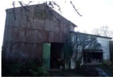
Figure 2. The northwest elevation of Barn 1
