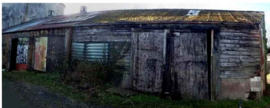
Figure 9. The northeast elevation of Barn 3.
