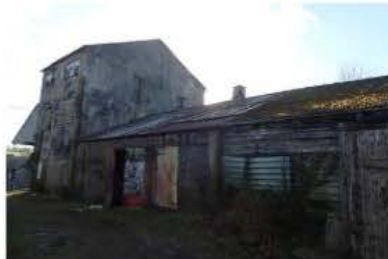
Figure 4. The northeast elevations of Barn 3 (in foreground) & Barn 4 (in background)
