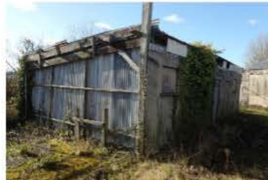
Figure 5. The northeast and southeast elevations of Barn 6
