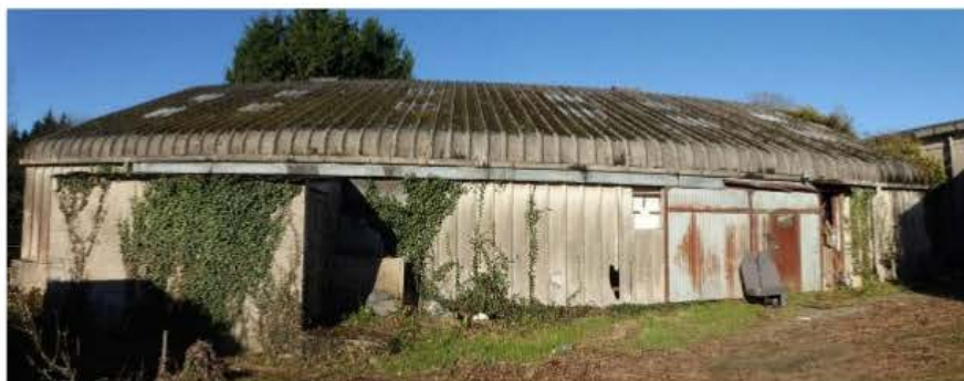
Figure 8. The southeast elevation of Barn 2.
